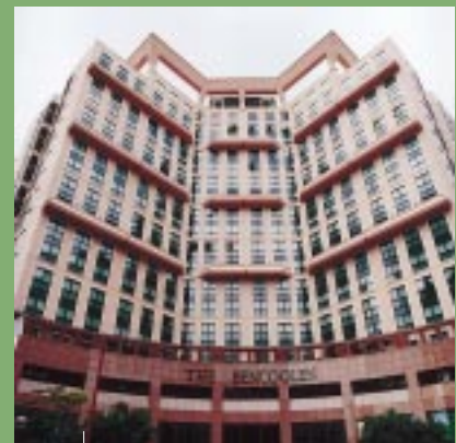
The Bencoolen- Condominium
